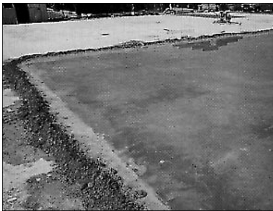
Figure 6: Ponding method of water curing
